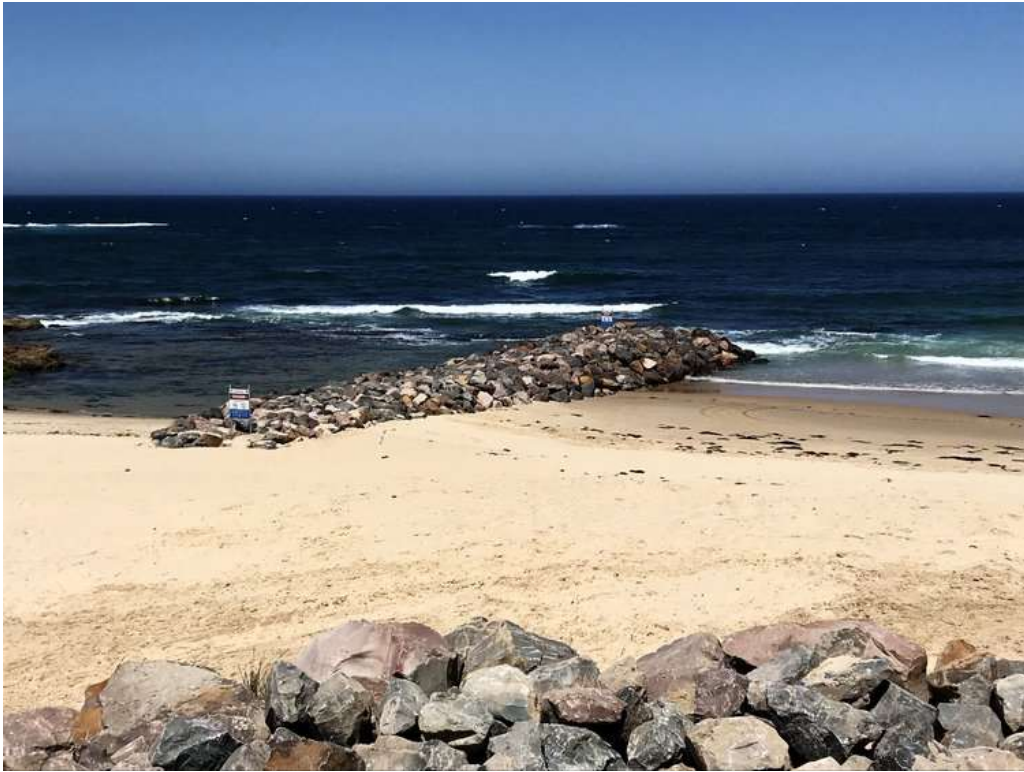
拋石式突堤(rubble mound groin(jetty))
